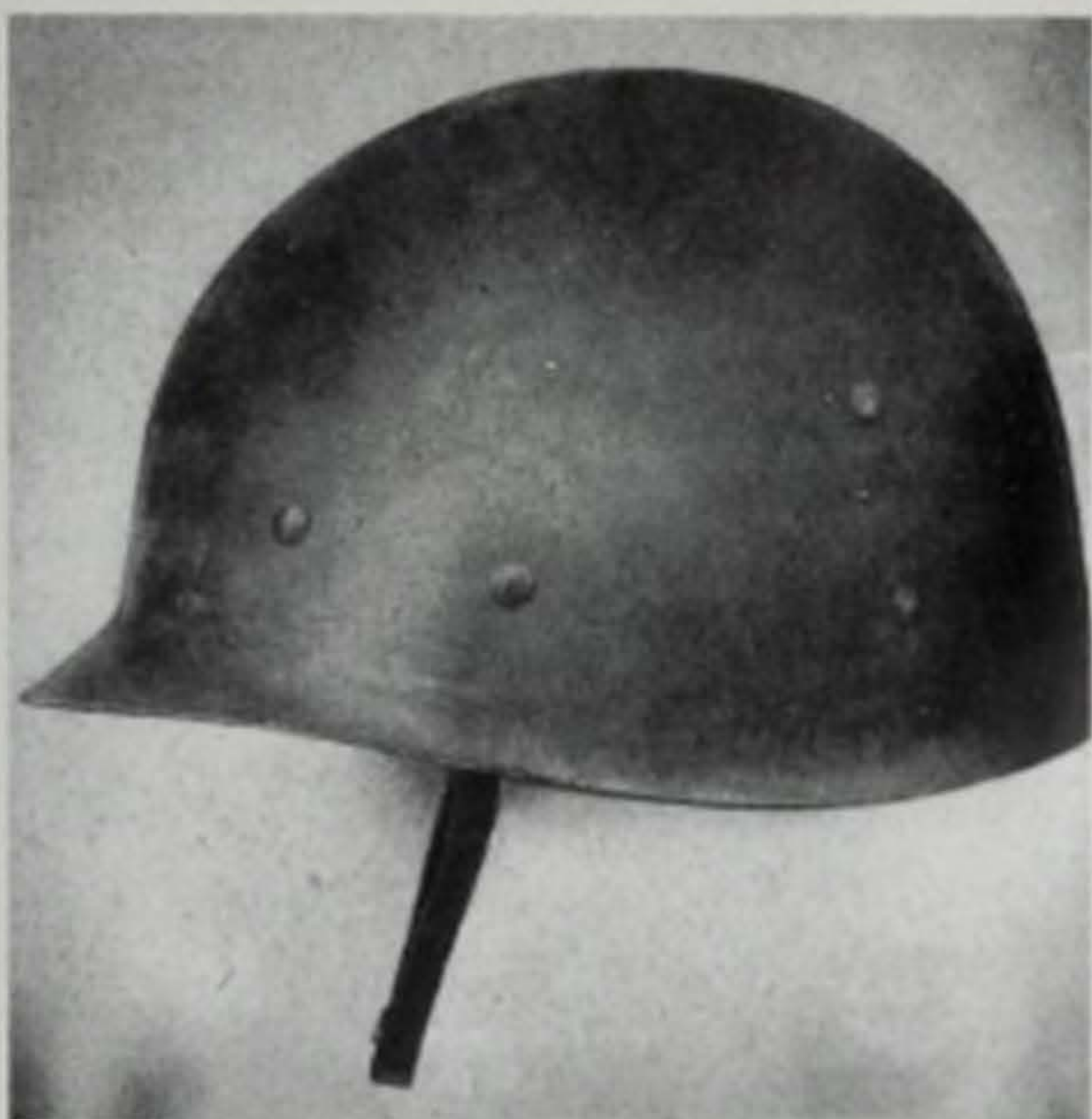
Exterior view of M-1 plastic helmet liner, ca. 1942. (Courtesy of U.S. Army Ordnance Department via National Archives, RG 156 Ordnance.)
