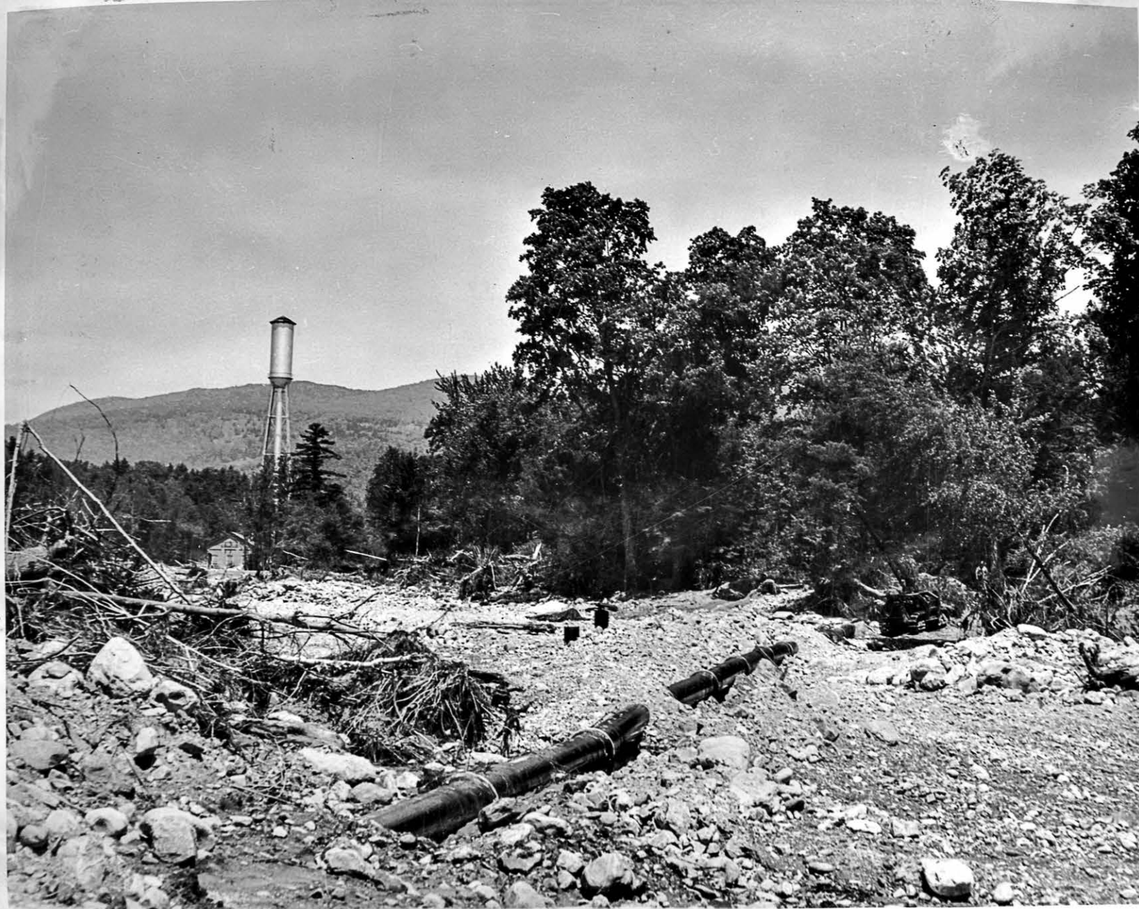
A view of the city reservoir. It is a complete loss along with 720 feet of pipe. Total damage here was around 50,000 dollars.
