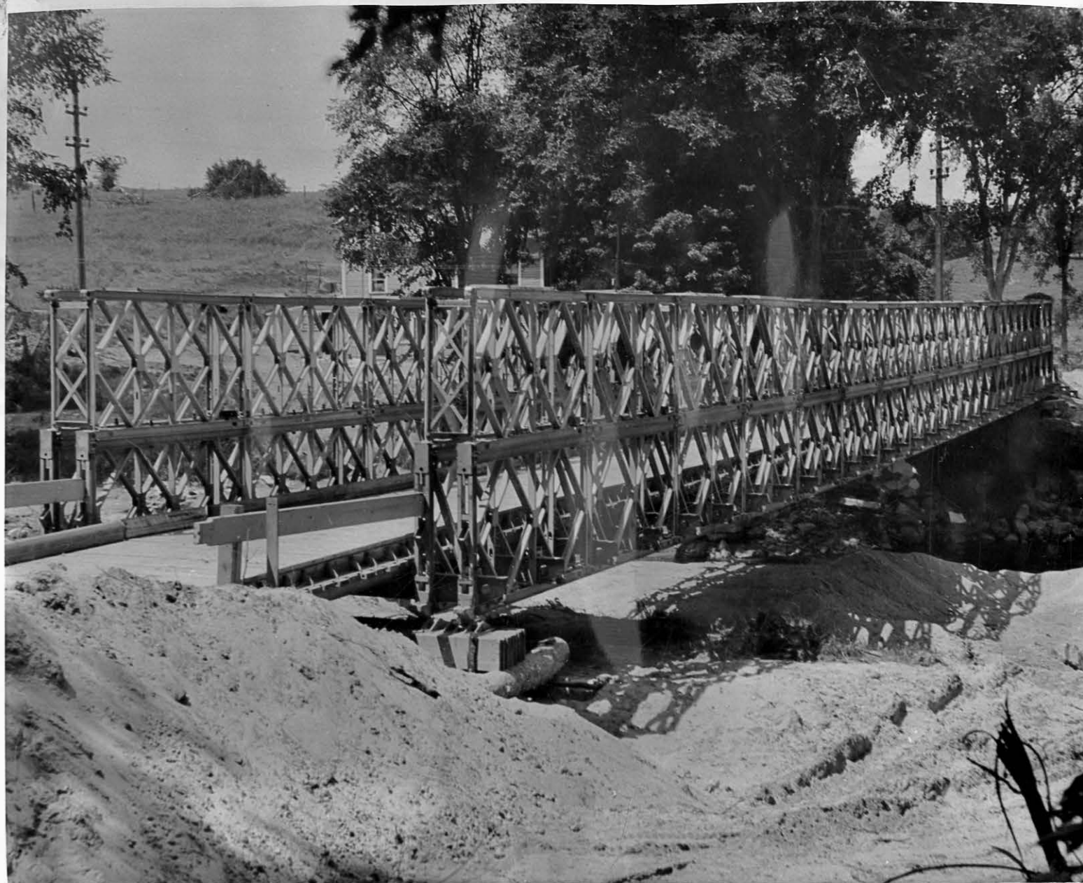
This Army Bailey Bridge soon took the place of the temporary bridge. Total amount of damage to Mill Village was estimated at $100,000.
