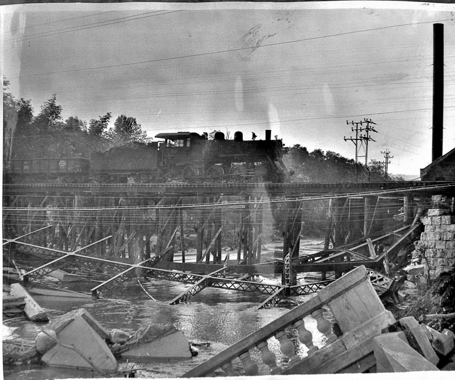
The temporary railroad bridge which has been constructed on wooden pilings. (Cost: $18,000)
