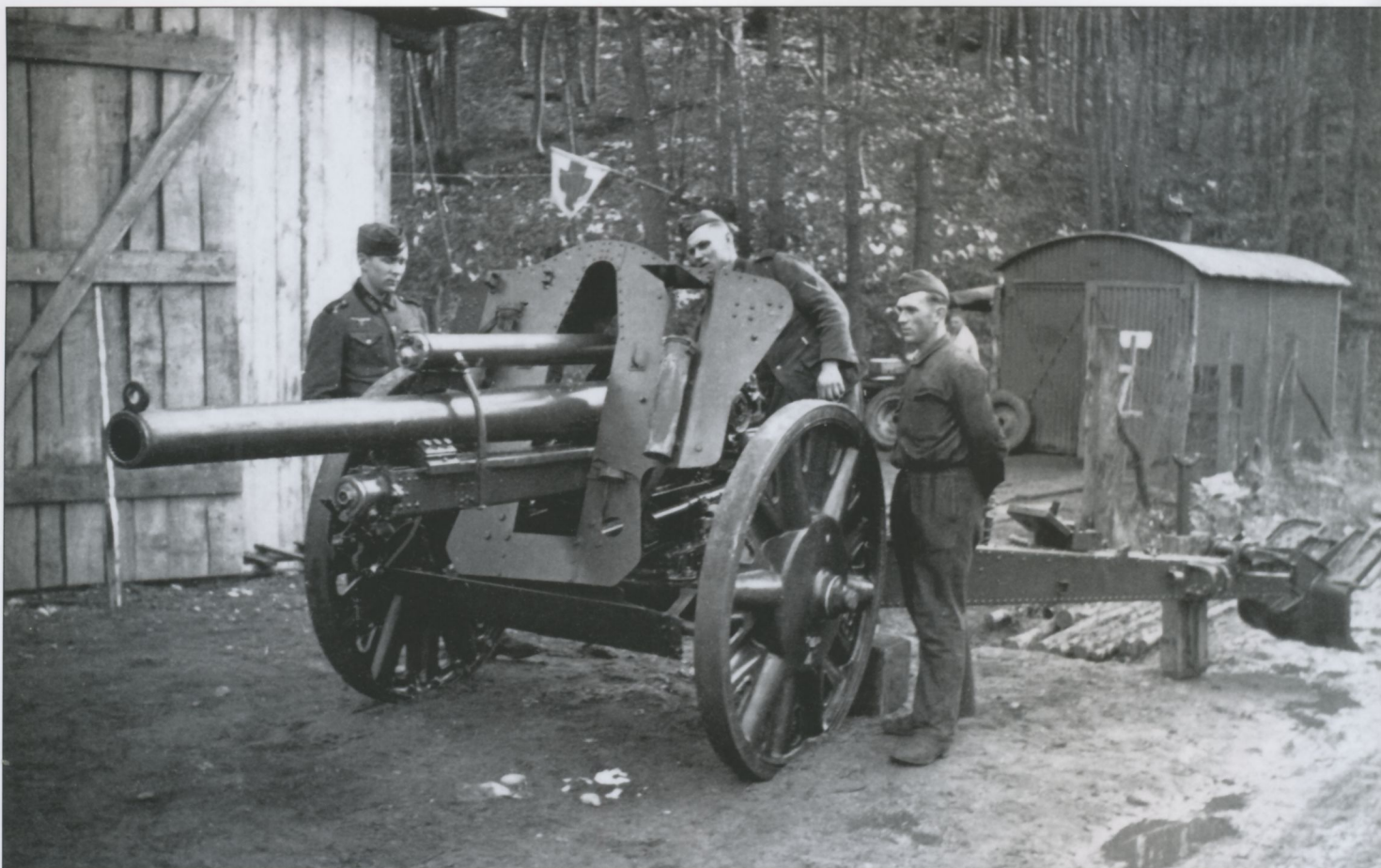
A 10.5cm IFH18 light field howitzer. This leichte Feldhaubitze is fitted with the rubber rimmed steel wheels intended for towing by trucks or halftracks. The "18" in the howitzer's designation does not represent a year model as later weapons, but a post-World War I series designation. It was developed in the late 1920s and made the standard field artillery piece in 1935. This weapon is in the process of being bore-sighted, that is, the sight aligned with the gun's bore for use when using direct fire.
