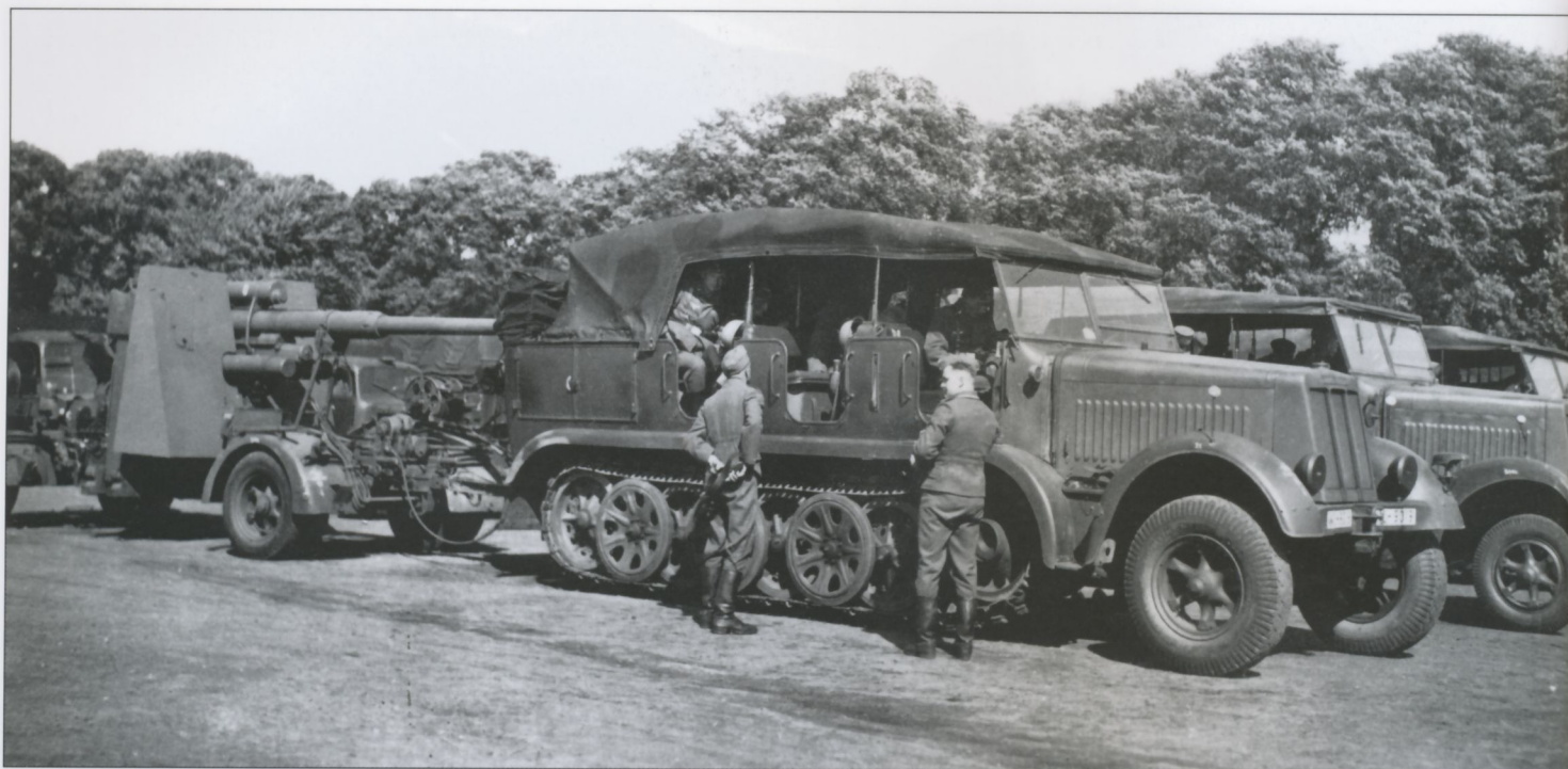
A Luftwaffe 8.8cm Flak 36 gun in tow behind a 12-ton SdKfz 8 heavy halftrack. Note the halftrack's brown and green camouflage canvas cover. Luftwaffe Flak troops wore blue gray uniforms with red collar tabs and red piping on their shoulder straps.
