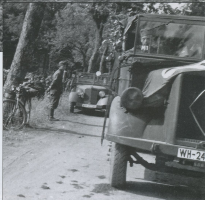
A 5-ton heavy cargo truck tows a Magirus motor bus (Kraftomnibus) out of the mud at a stream crossing ford. Buses, while certainly not cross-country vehicles, proved valuable to carry troops and equipment. Limbs have been laid as a crude corduroy road to prevent vehicles from bogging down on the muddy shore.
