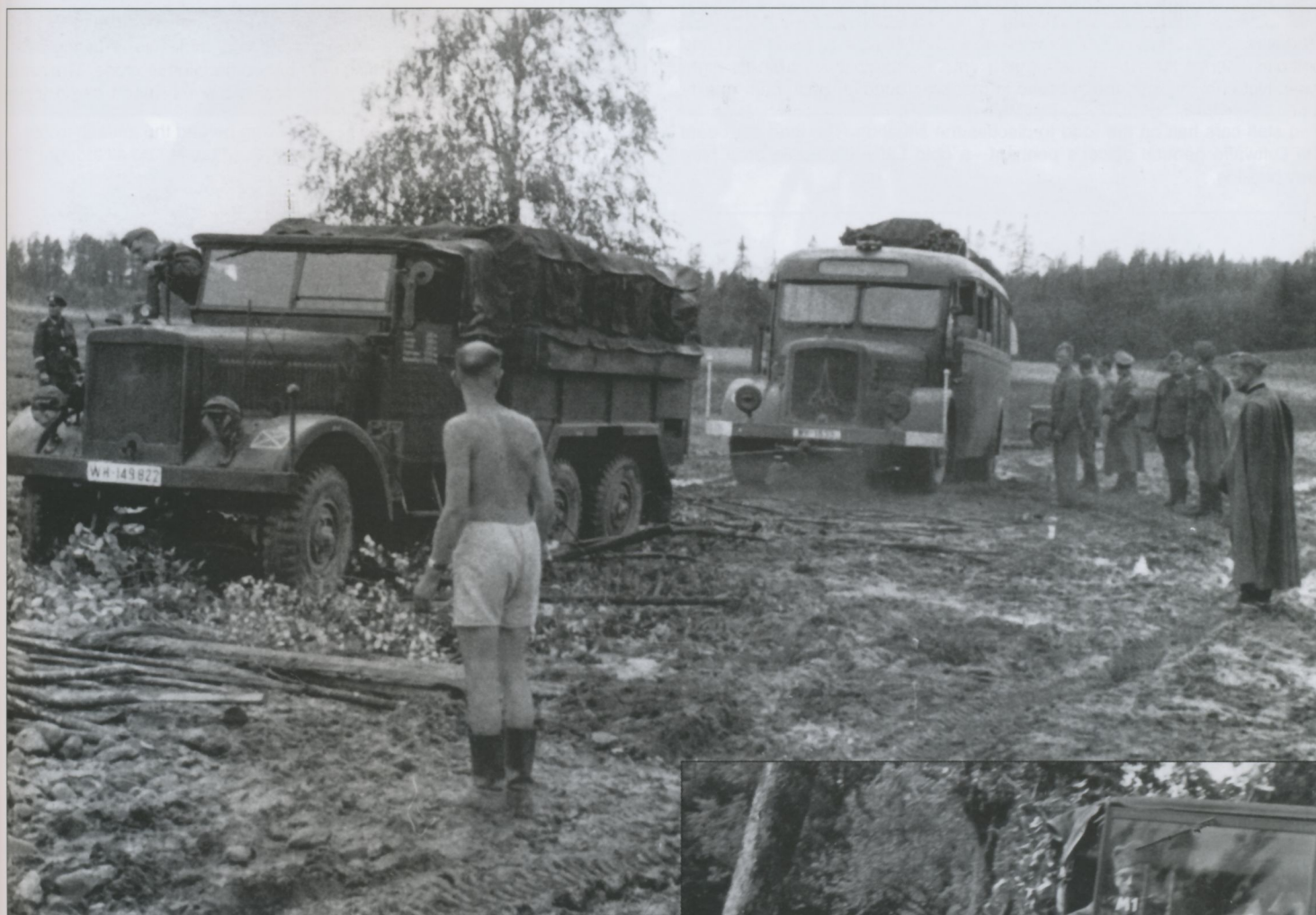
A 5-ton heavy cargo truck tows a Magirus motor bus (Kraftomnibus) out of the mud at a stream crossing ford. Buses, while certainly not cross-country vehicles, proved valuable to carry troops and equipment. Limbs have been laid as a crude corduroy road to prevent vehicles from bogging down on the muddy shore.
