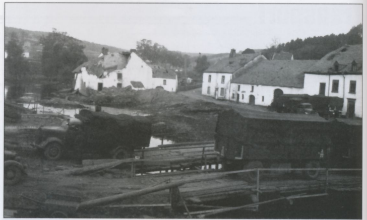
In a shell-battered town two side-by-side bridges have been built to allow two-way traffic. Often only one-lane bridges were available requiring traffic controllers to alternately allow traffic from either direction to cross. The cargo truck is towing a 5-ton E5 standard trailer. This widely used cargo trailer could carry a 5,000-kilogram payload.
