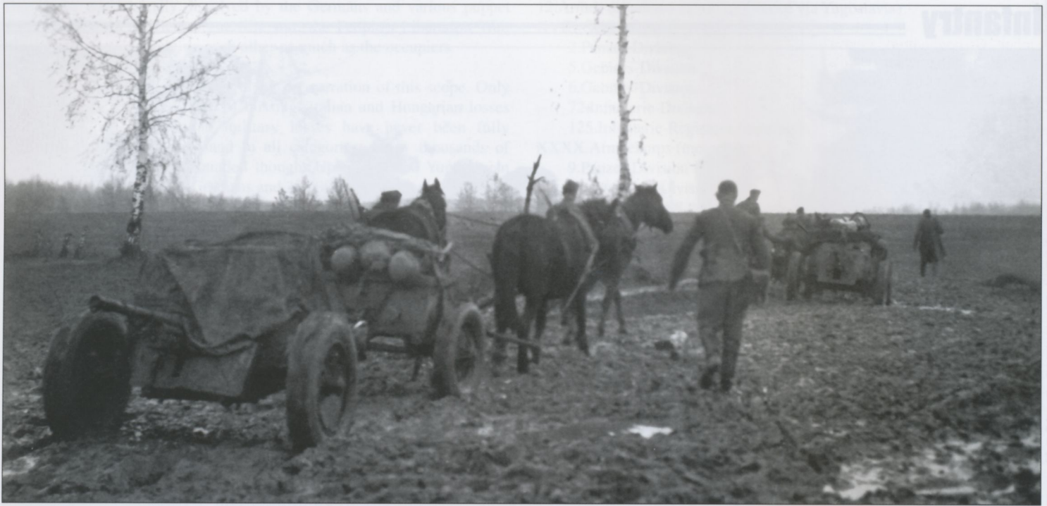
2.Armees drive from Austria. A 3.7cm Pak 35/36 antitank gun and its SdAh 32 ammunition limber (with fenders removed) are drawn by a team of horses with a third added because of the mud. Even in infantry regiments light trucks were normally provided to move antitank guns, but many recently raised infantry divisions and mountain divisions relied on horses. Motorized prime movers were preferred as it was necessary to rapidly relocate antitank guns from position to position in order to survive and effectively engage tanks. Note the crew's helmets slung on the limber.
