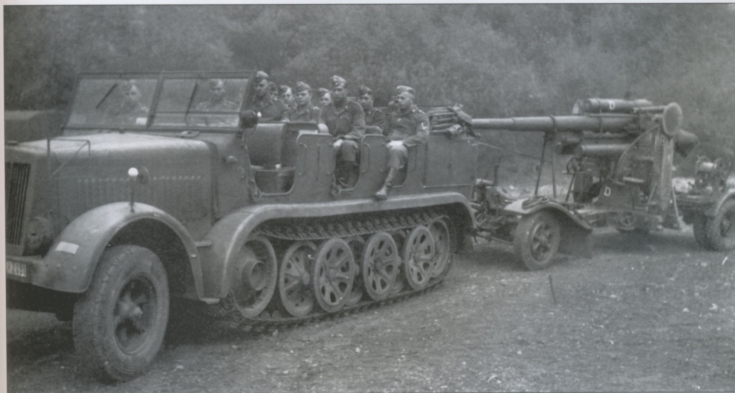
A Luftwaffe 12-ton SdKfz 8 heavy half-track tows an 8.8cm Flak 18 gun, what they called the "Acht-Acht." Note the white "D" painted on the gun mount and recoil cylinder. A battery's four guns were designated A to D and this was often marked somewhere on the weapon. Army artillery batteries followed the same practice. Verbally they were referred to by their phonetic alphabet letters: Anton, Bertha, Cäsar, and Dora.
