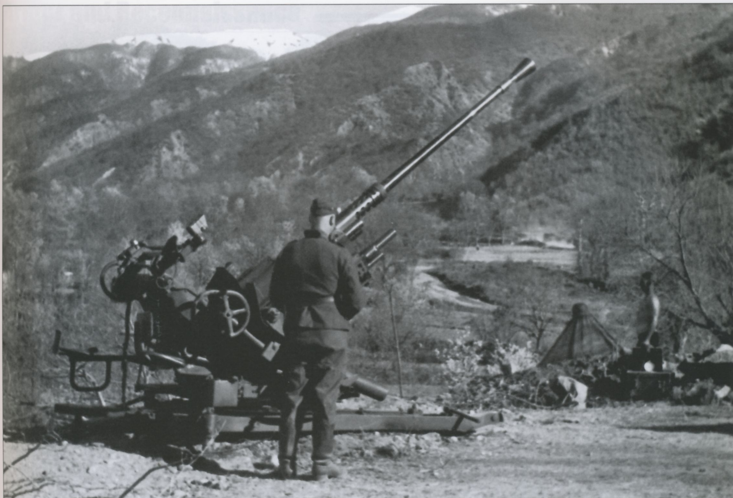
A 3.7cm Flak 36 anti-aircraft gun set-up in an unprotected position on the Yugoslavian-Bulgarian border. It was normally towed on a two-wheel carriage. A few of these guns were assigned to light Flak battalions while the bulk of the battalion's guns were 2cm weapons. The 3.7cm offered about a third more range than the 2cm, but with a much slower rate of fire; 80 rounds per minute as opposed the 2cm's 700-800 rounds per minute. Note the steel helmet atop the Zeltbahn tent for waterproofing.
