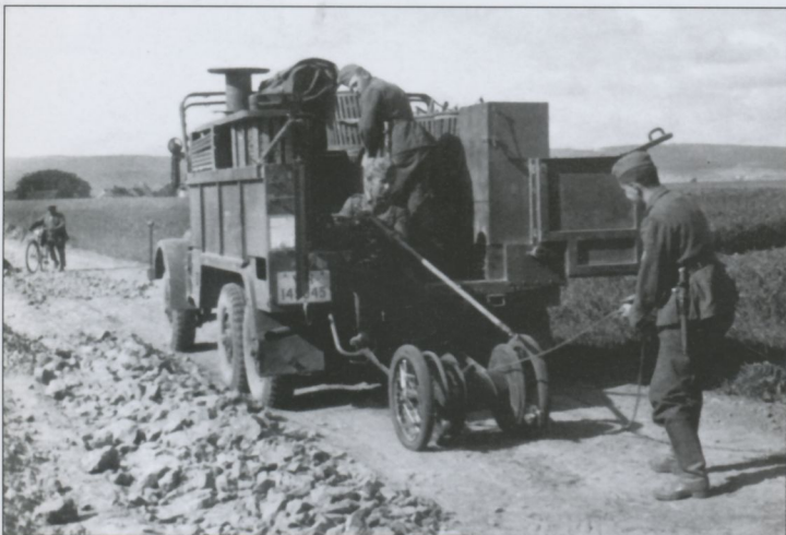
A field telephone cable truck (Feldfernkabelkraftwagen) tows a small cable reel as it strings telephone cable. This type of reel could be drawn by hand or behind a bicycle. Stowed in the back of the truck and on side racks are sectional poles used for temporary poles. For speed and when wire would be laid for only temporary use it was simply laid on the ground. This though made it susceptible to breakage by friendly vehicle traffic.
