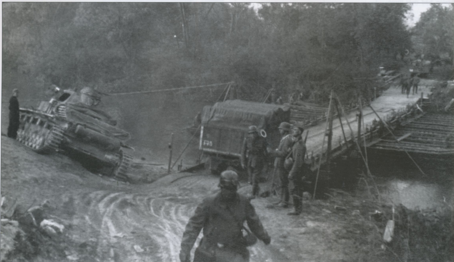
Rivers, streams, gullies, and gorges were widespread in the Balkans keeping the pioneer troops gainfully employed. Here medium pontoons boats (Brückengerät T) are used to span a large stream by XIV.Armeekorps (motorisiert) as Feldgendarmerie (field military police) direct traffic. The parked PzKpfw IV has probably suffered a mechanical breakdown, a common occurrence on a road march.
